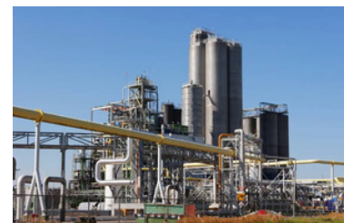
Chemical industrial park
